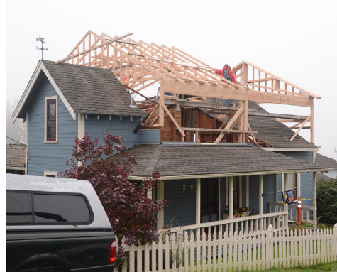
ALL ROOF TRUSSES UP, OCTOBER 18, 2013
