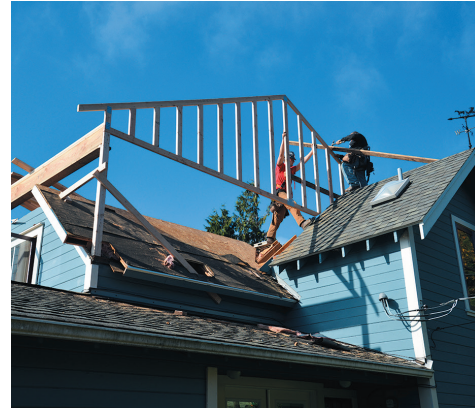
TRUSS ERECTION SHOWING ROOF TEAR-OUT, OCTOBER 17, 2013
